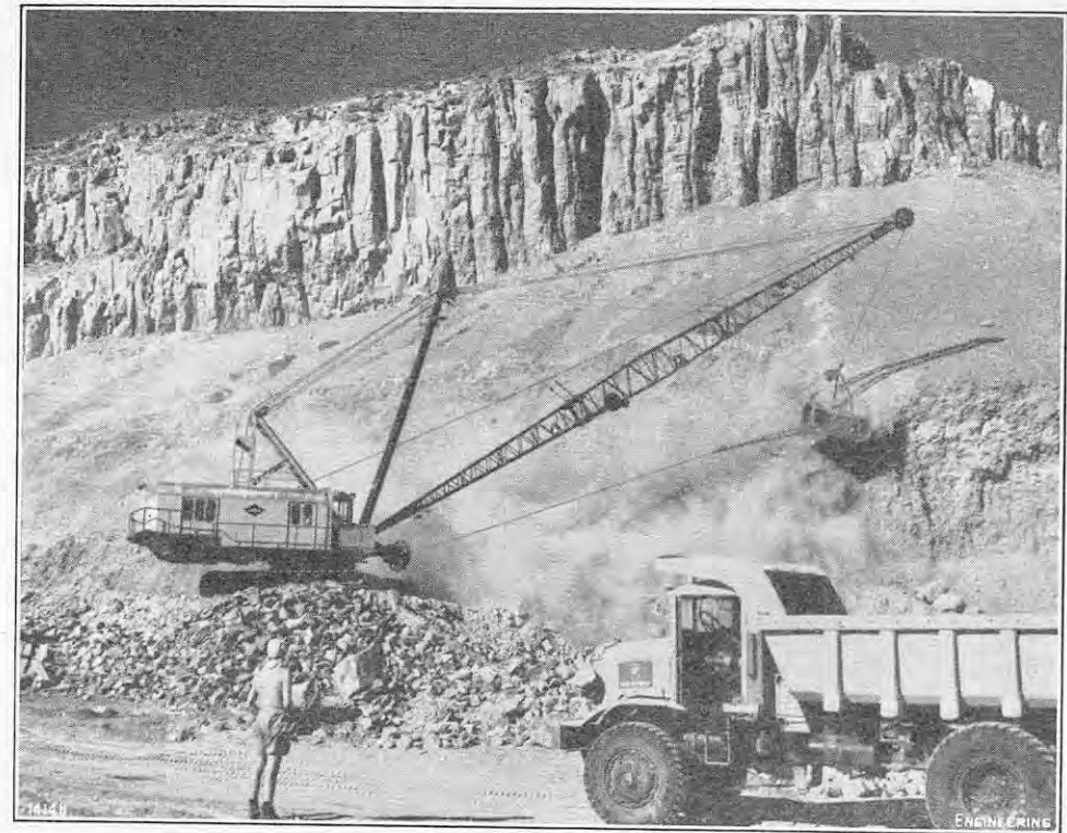
FIG. 2. WORK AT A QUARRY FACE.
