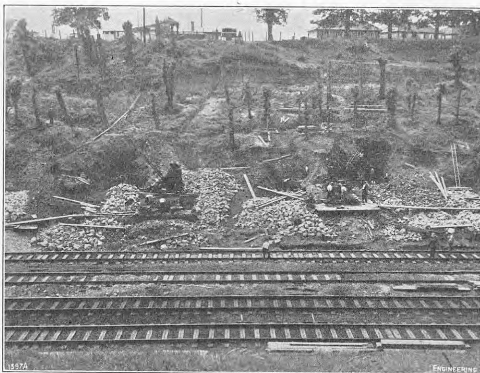
FIG. 6. SLIP AT SONNING CUTTING.
